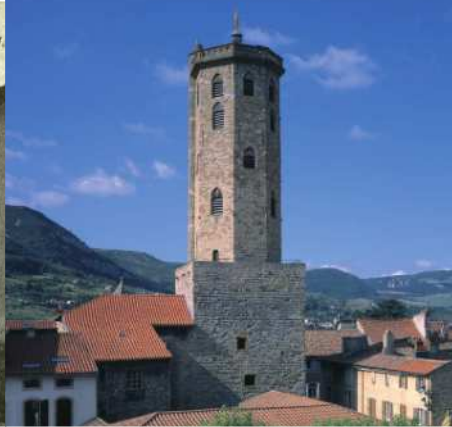
The tower of the kings of Aragon viewed from the south, on top of which sits the polygonal tower, was a symbol of the domination of the kings of Aragon towards the end of the 12 th century.
