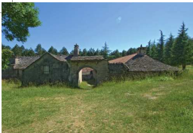
Les Cades Farm is built around a yard comprising a house and two long vaulted sheepfolds, one of which contains a bakehouse with a limestone lauze roof.
