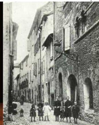
This mediaeval house at 55 rue Peyrollerie may have lost its gemel windows and decorative cordon but it has kept its large shop arcades on the ground floor.
