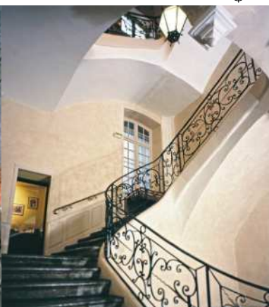
The staircase of the hôtel de Pegayrolles with its wrought iron balustrade, characteristic of the 18 th century in Millau.
