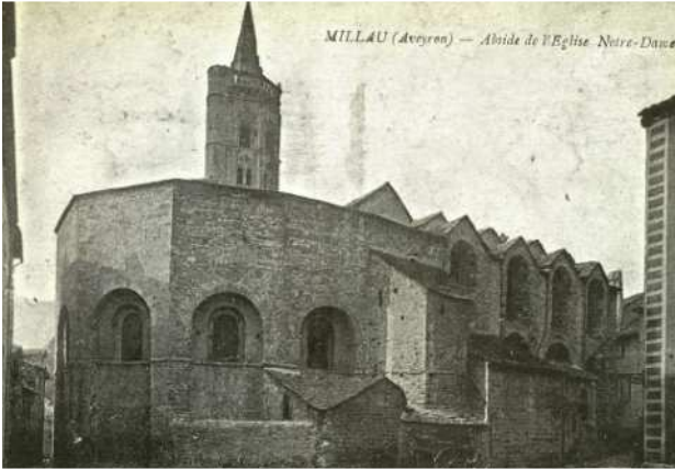
The polygonal chevet of the church and its northern elevation, next to which can be seen the chapels which were added, and then destroyed, in the 19 th and 20 th centuries.
